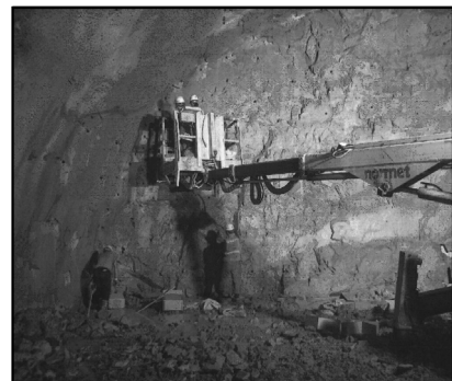
Fig. 16. crown test point setting
