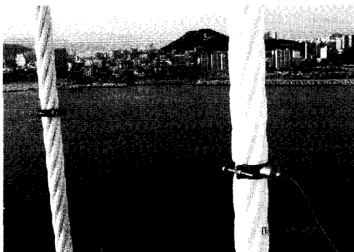
〈Fig. 9〉 Accelerometers installed at hanger cables
