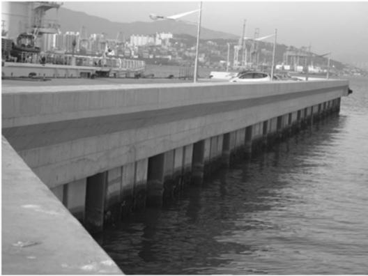
Fig. 1. Breakwater with perforated vertical wall.
