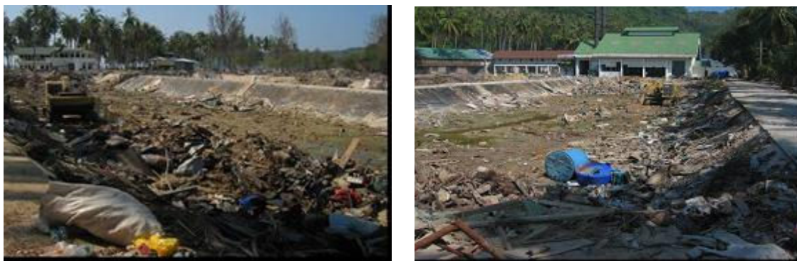
Fig. 3. Damages of wastewater treatment systems on Phi Phi Island
