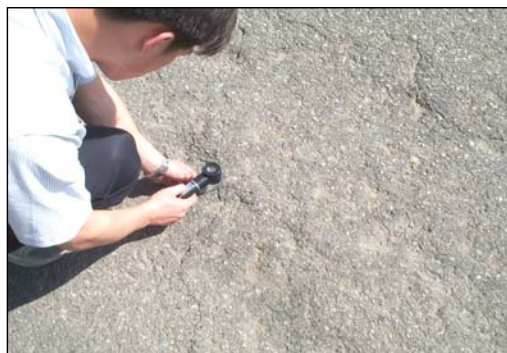
FIGURE 5. Crack measurement using crack gage
