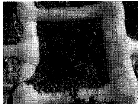
Fig. 3. Geotextile Flexible Crib
