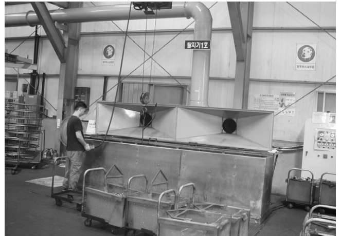
Figure 4. A case on the semi-automatic degreasing work using crane by open top degreaser
