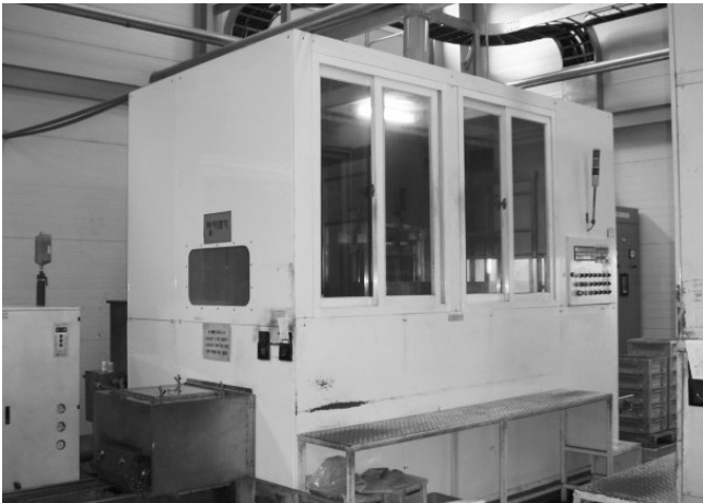
Figure 3. A case on the automatic degreasing work by an enclosed system
