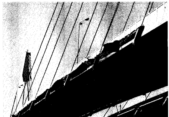
Fig. 4. Picture of Jin-do bridge after collision.
