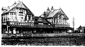
Fig. 1. YongSan Railway Station on the Kyungui Line 3)
