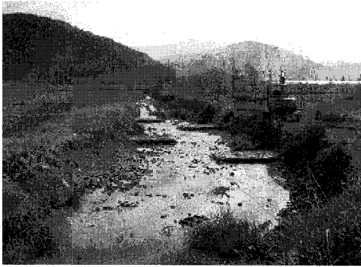
(a) just after construction(2004)
