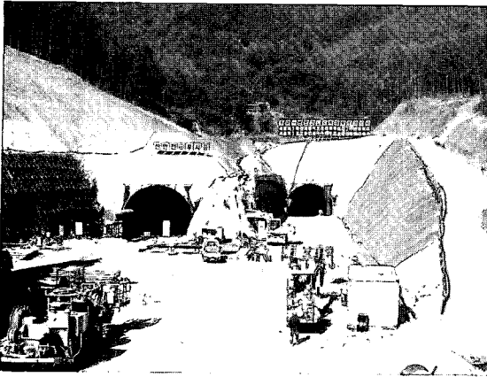
Fig. 2. Field test at Gyea-Ryong tunnel.
