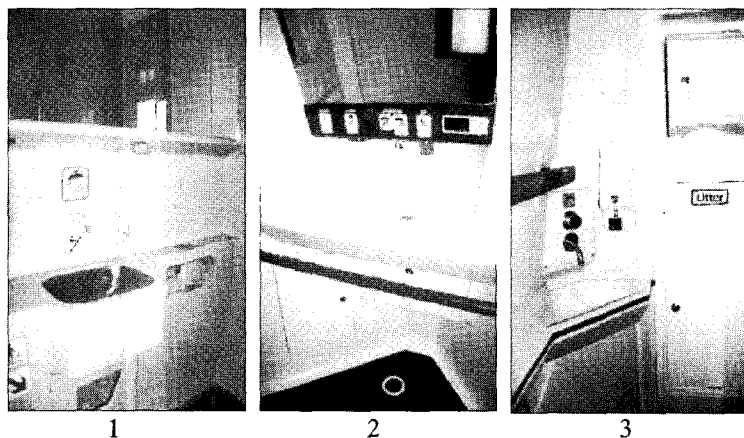
Fig.6 Built-in appliances unit system 1:ICE(Germany) / 2:Euostar(Italy) / 3:SNCF(France)
