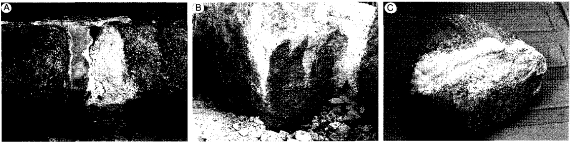
Figure 3. The production status of efflorescence caused by cement. (A) Transformed layer of ash color caused by cement through material. (B) White phenomenon caused by using excessive mixture. (C) Remaining material of lime grown like a stalactite.
