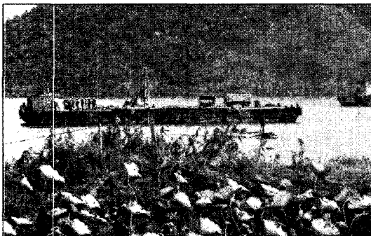
Fig. 3 Drilling work using a barge
