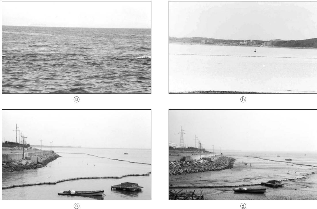
Fig. 1. Examples of silt protector in the west coast of Korea
