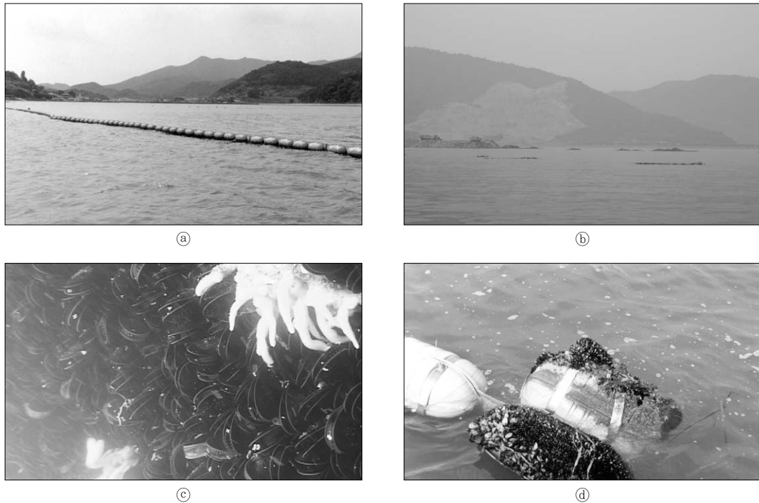
Fig. 3. Examples of silt protector in the south coast of Korea
