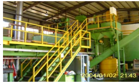
A Mechanical sorting with Hoods installation
