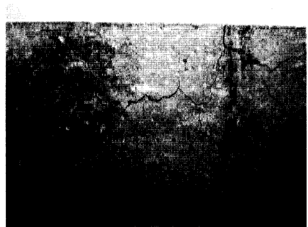
Fig. 12 Cracks caused by the alkali-silica reaction of the crushed stone used in the experiment.
