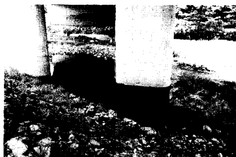
(a) Pier tested
