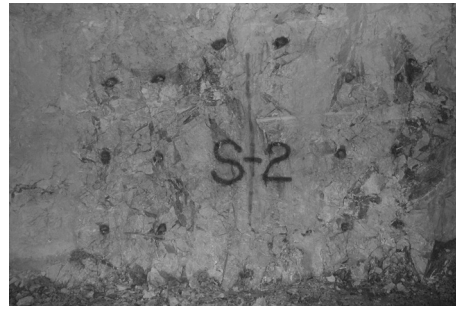
Fig 7. Blast design scheme (Cylinder-cut, V-cut wedge)
