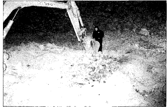
Fig. 14. Dump loading of rocks by excavator
