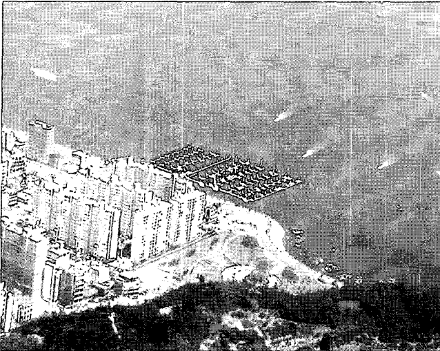
Fig. 4 Application of floating type marina.
