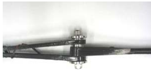
Photo.1. End part connection of U anchor type.
