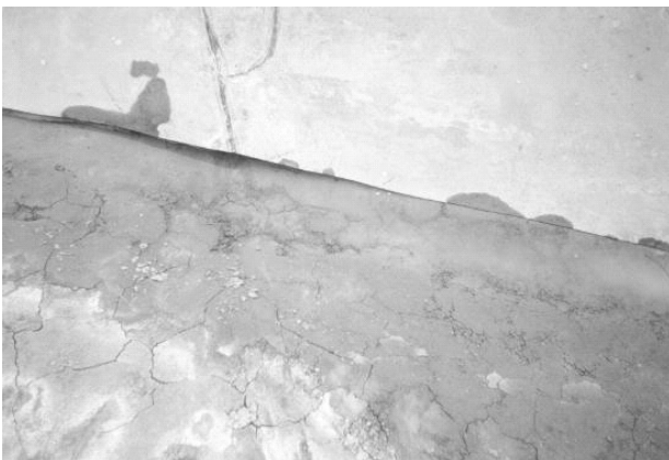
Fig. 3. Close-up of hydrated bentonite accumulated on top of geomembrane on cell base after removal of overlying sacrificial geomembrane.
