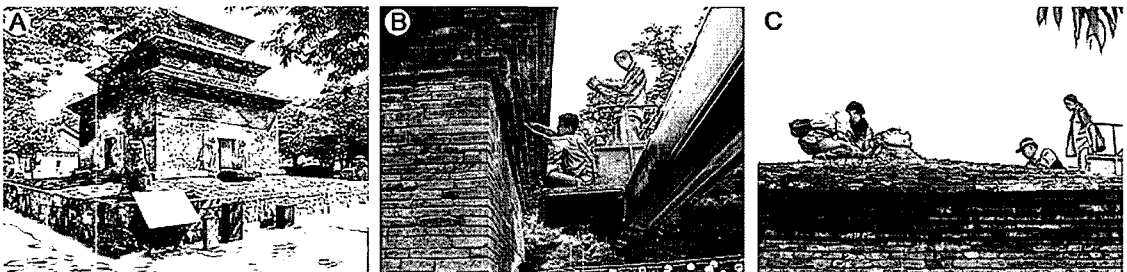
Figure 1. Field occurrences of the stone pagoda in the Bunhwangsa temple. General view of the southwestern side (A). Stalactite-like white grey precipitates collected from northern body rocks of the pagoda (B). Photograph shows detail survey in the uppermost roof of the 3rd floor (C).
