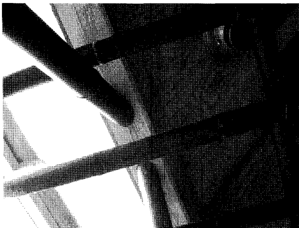
〈Fig. 15〉 Round bamboo-boxed beam connection with the bamboo connector with the bamboo connector in the passageway in the passageway
