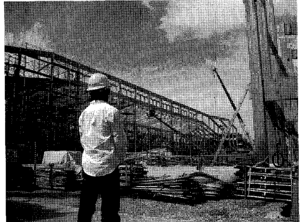
〈Fig. 17〉 Under construction (Main exhibition hole before assembling of roof)
