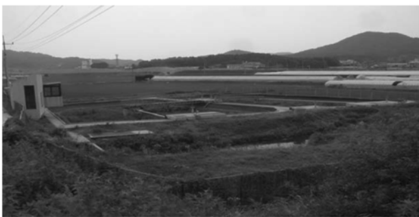
Fig. 4. Photographs of subsurface-flow wetland facility.
