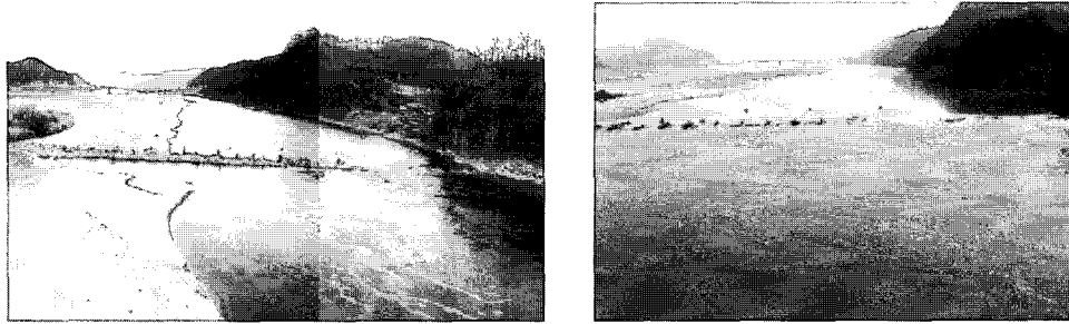
Photo. 1. Section control by dike located in distant 300 meter from Gongju gauging station
