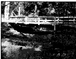
(b) Original Bridge image
