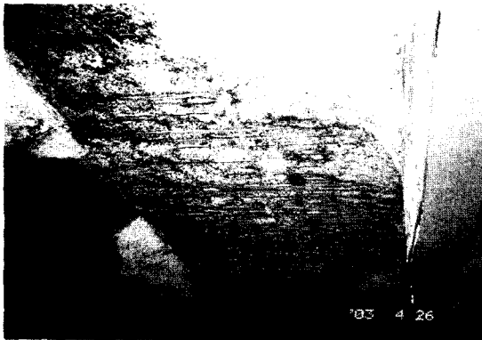
(b) Concrete exfoliation and exposure of reinforcing bars
