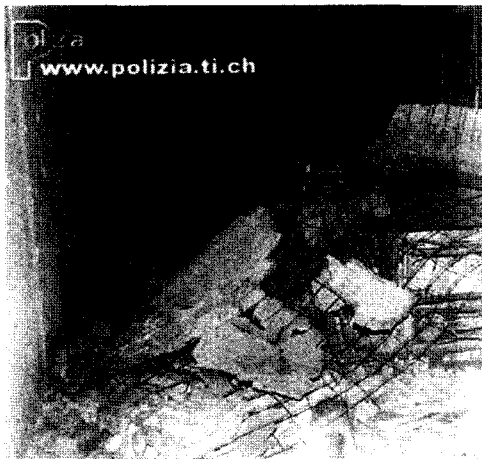
Fig. 3. Sectionally collapsed false ceiling in the Gotthard tunnel(after Haack, 2004)
