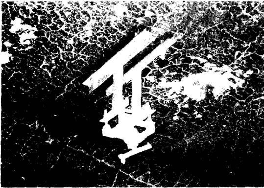
(a) Thermal cracking
