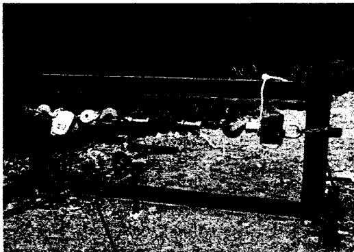
(b) 폴리머애자 (Polymer insulator)
