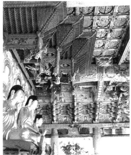
Fig. 2. The Inside of main building shown in Fig. 1.
