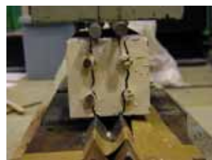
Figure 6. Operation to take out the rebar from the concrete.
