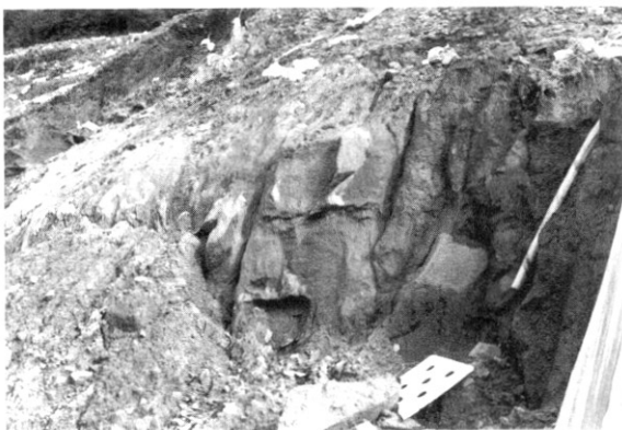
Figure 5. Landslide of Diollite area.
