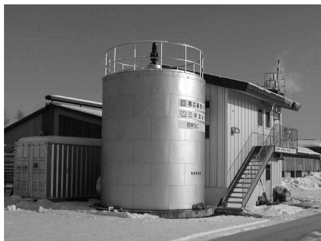
Figure 12. Biogas model plant in a farm attached to Obihiro University.
