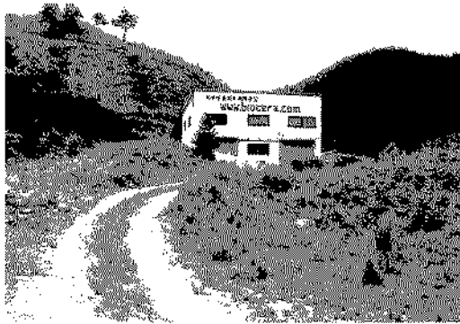
Fig. 1. A view of the Samsung mine area.
