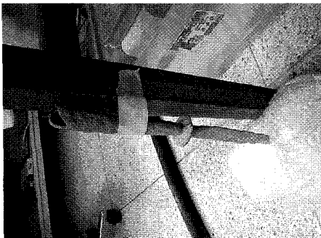
Fig.11. reinforcing inside of model with reinforcement.
