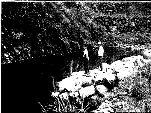
Photo 5. Concrete Deflector with Rock Coating
