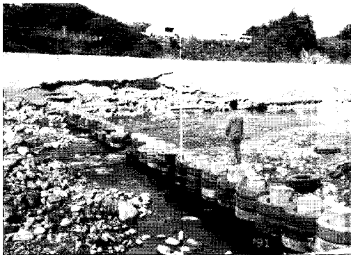
Photo 3. Tire weir with opening
