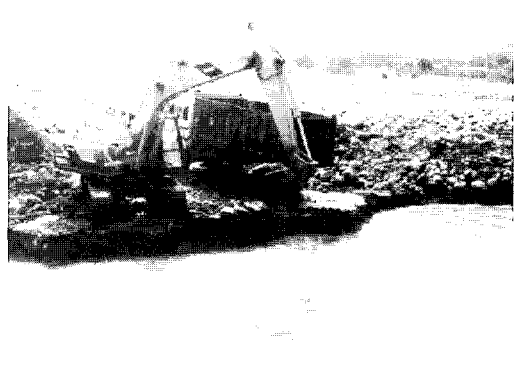
Photo 4. Channel Excavation
