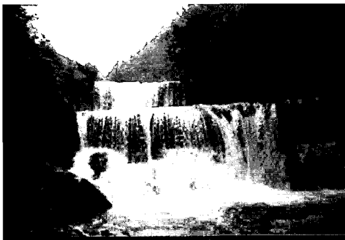
Picture 7. Dam No.1 (April, 2000)
