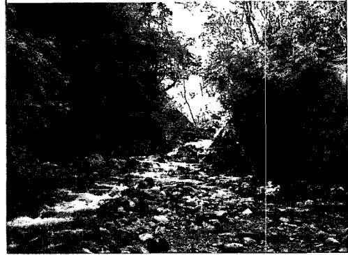
Picture 4. Dam No.3 (November, 2000)
