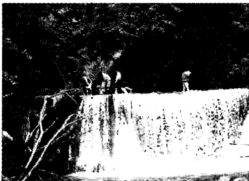
Picture 1. Dam No.4 (April, 1999)
