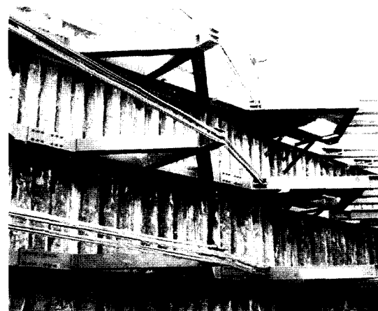
Photo 2. IPS wales in urban excavation
