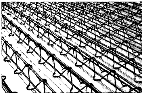
Fig. 1 Deck plate system with lattice bars
