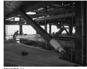
FIGURE 11 TAYLOR DAMPER INSTALLATION, SHORT WALLS
