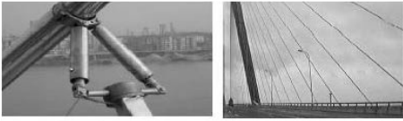
a. Dongting Lake Bridge
