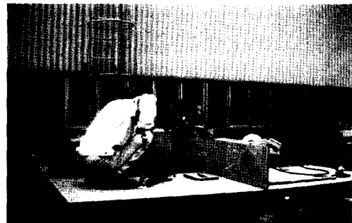
Fig. 3 Forced fit-up for alignment before welding
