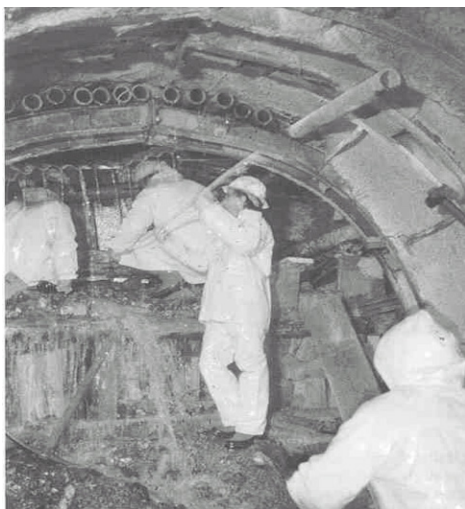
Fig. 9 Forepoling insertion ahead the TBM (Salvi Penati, 1991)
