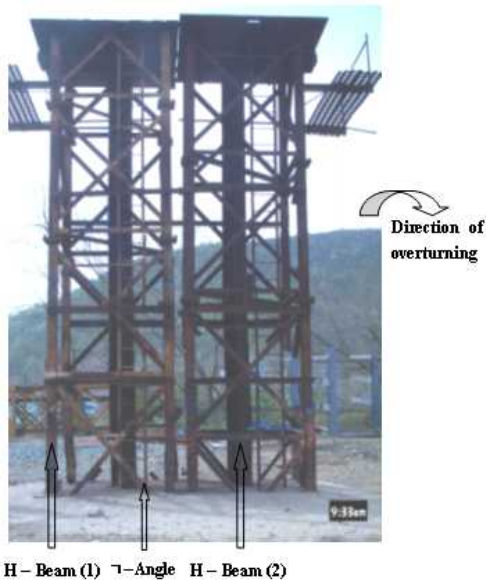
Fig. 7 View of the steel structure
