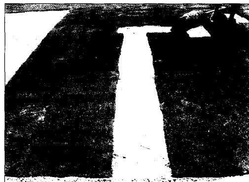
Fig. 2. Sodding by roll sod.
