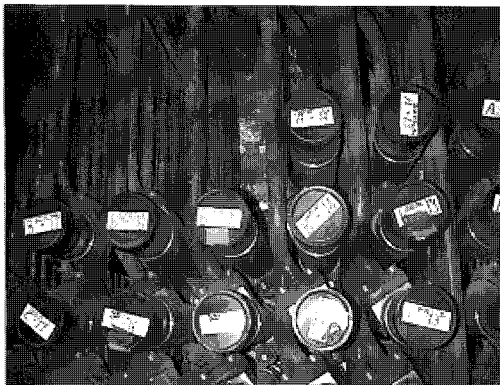
Fig. 1 Feeder pipes in pressurized heavy water reactor
