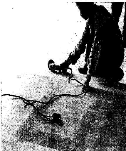
< Fig. 4 > Grinding operation by the hand
