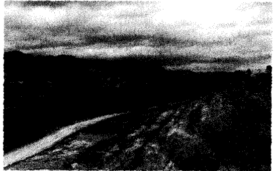
(b) View of stabilized slope
