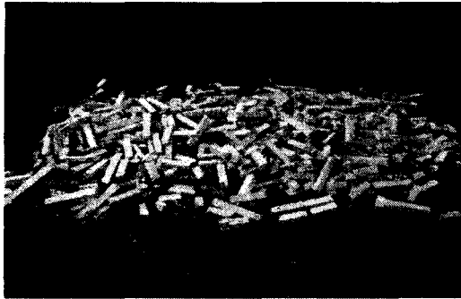
Fig. 6. Result of blasting demolition for scaled model #1.
