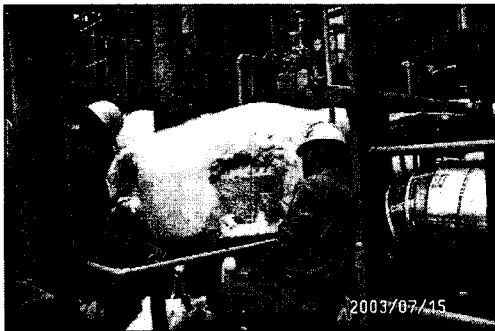
Fig. 4. Measuring vibration of secondary pump.
